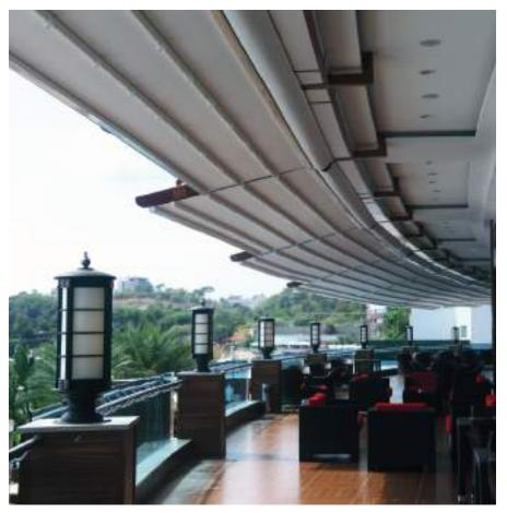
A suspension system project in a circular form for Granada Hotel, providing maximum shading and realized without using any pillar.
